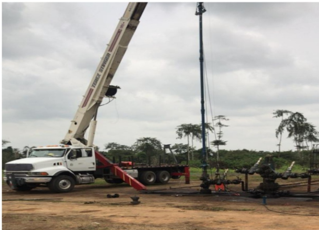
Pressure Control Rigged-Up on Tubing for Completion Operations
